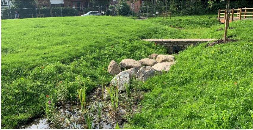
Figure 14 - Main swale and check dam flow control feature
